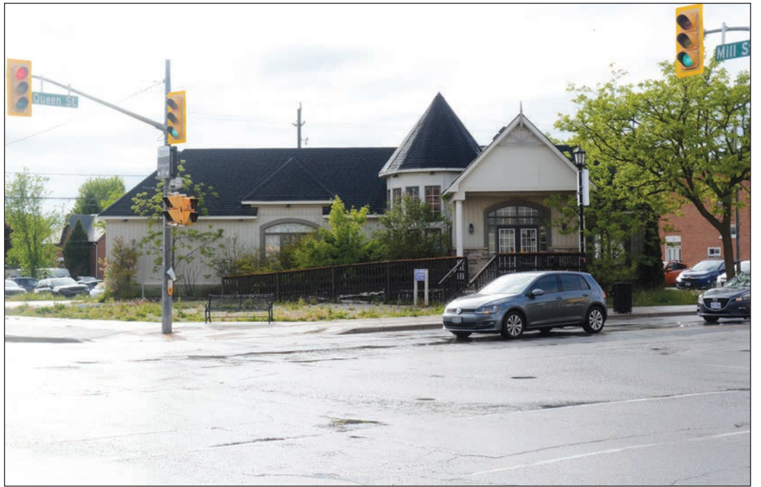
ENHANCED PARKING – The Town of New Tecumseth has purchased six properties in downtown Tottenham with plans to create more parking. The current office space on the corner of Queen Street and Mill Street will be demolished to increase the number of parking spaces downtown.
